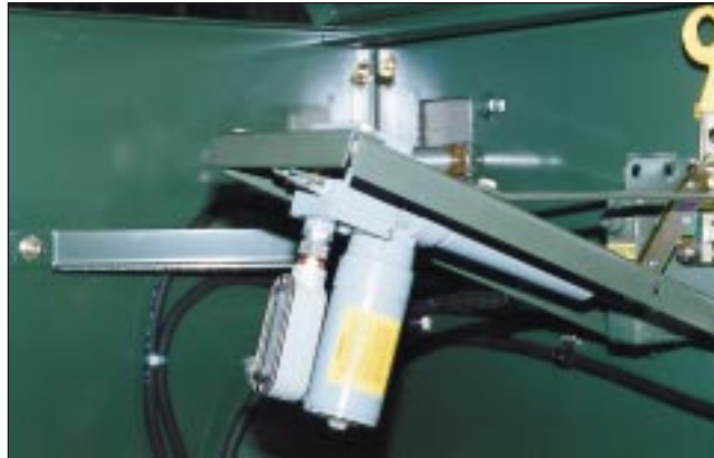
DC Motor Actuator - Connected.
